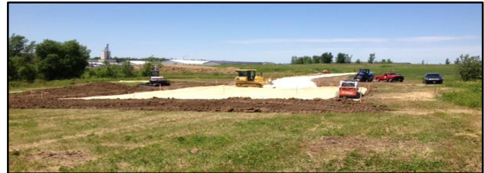
Work at Waldo's Rock Park begins.
