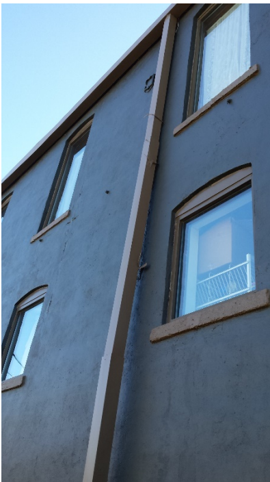
Patch and paint stucco at removed insulators
