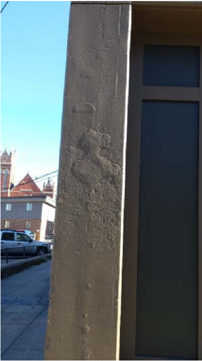
Improved patching complete. rePaint
