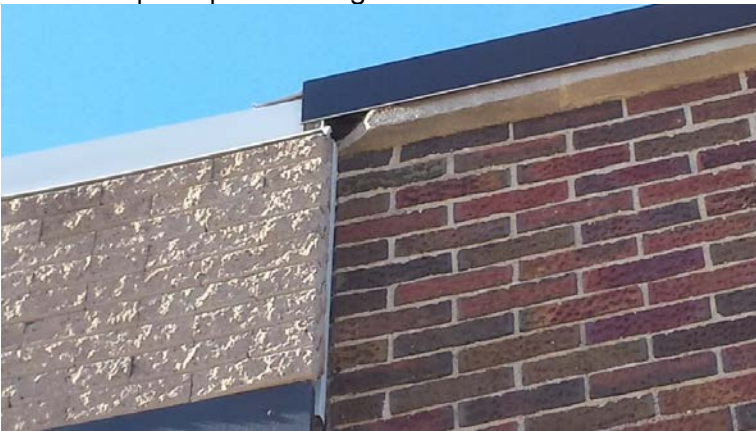
Fill/Repair stone cap per drawings
