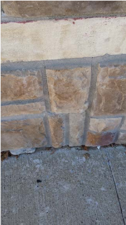
Repair cracks in stone veneer mortar Patch and paint per drawings.
