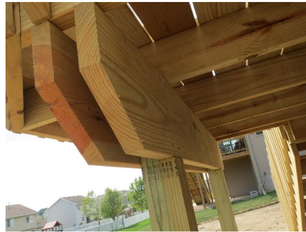
The support beam on the left is not supported by the 4 x 4 and was attached with nails. A 1/2" bolt through both support beams and the 4x4's are needed because if nails holding the beam fail the deck could fail.
