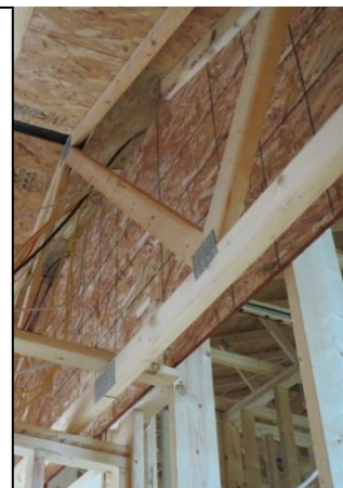
The support beam on the left is not supported by the 4 x 4 and was attached with nails. A 1/2" bolt through both support beams and the 4x4's are needed because if nails holding the beam fail the deck could fail.
