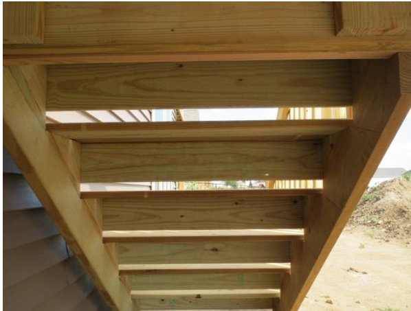
Deck boards can NOT span 36" without addition support in the middle of the stairs
