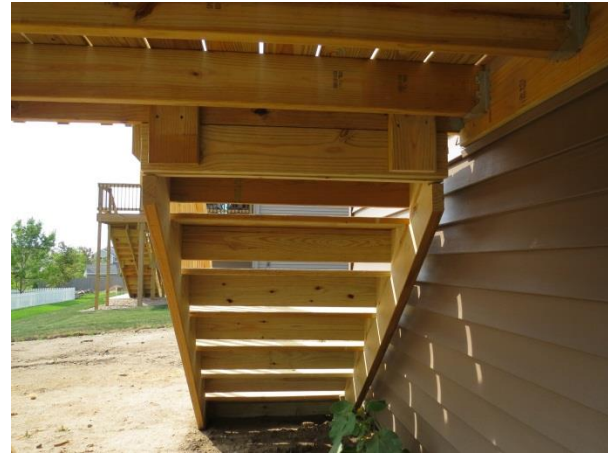
Deck boards can NOT span 36" without addition support in the middle of the stairs
