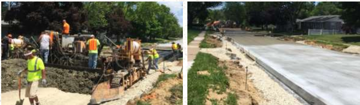
Hillview during pavement construction
