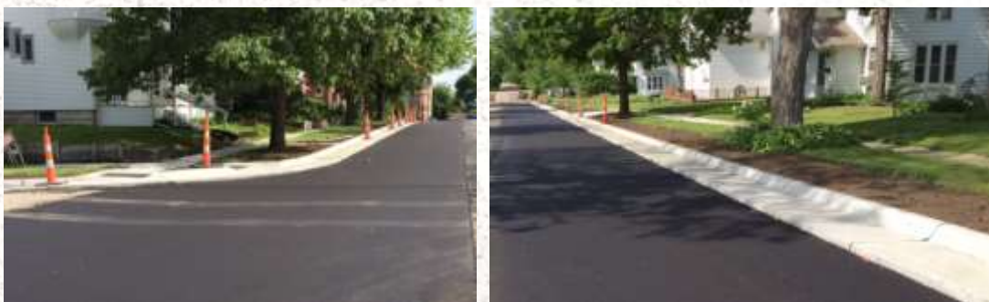
East side concrete work completed
