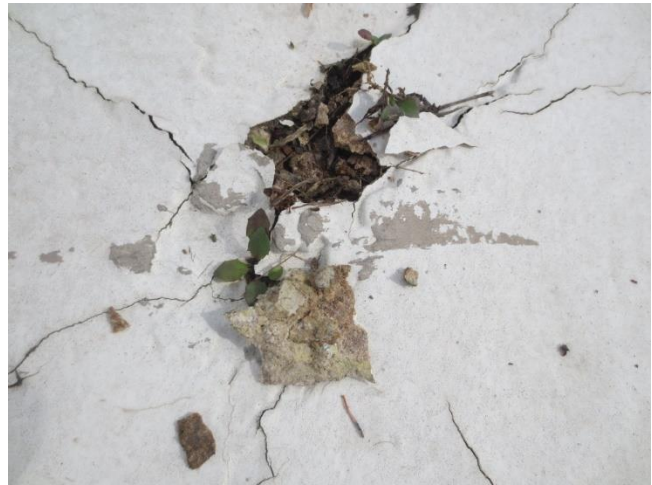
Concrete Failure – Pool Wall
