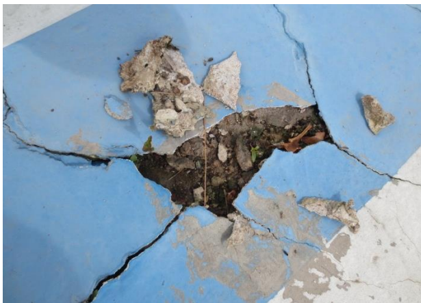
Concrete Failure – Pool Basin Floor
