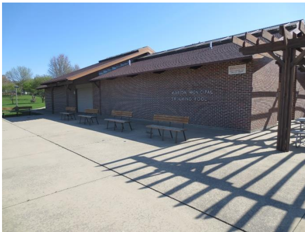
Entrance and Bathhouse
