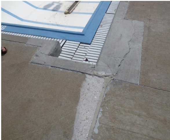
Concrete Failure – Pool Basin Floor
