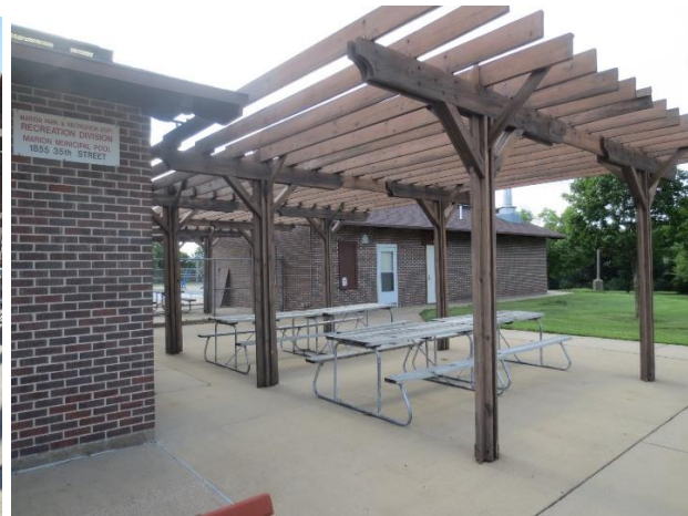
Outside Seating and Concessions/Mechanical Building
