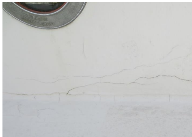
Concrete Failure – Pool Wall
