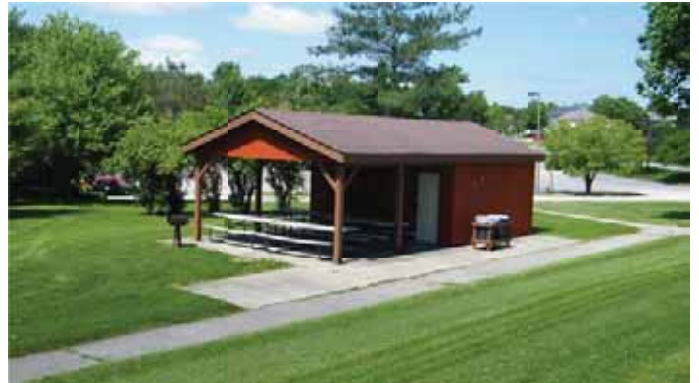
Image 2: Restroom facilities support extended user stays at both the pool and park.
