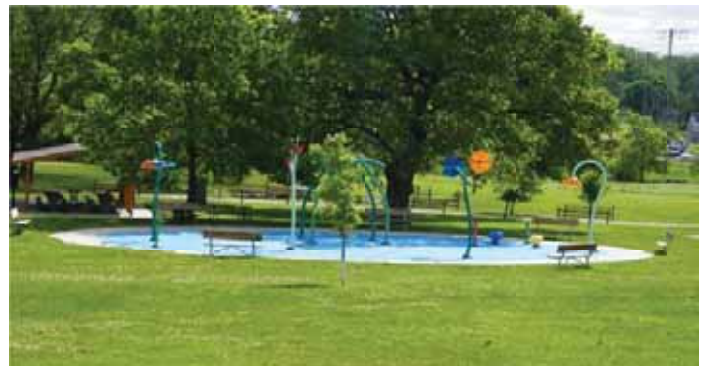
Image 8: New splash pad installation helps ease demand on the city aquatics facility and serve more residents.
