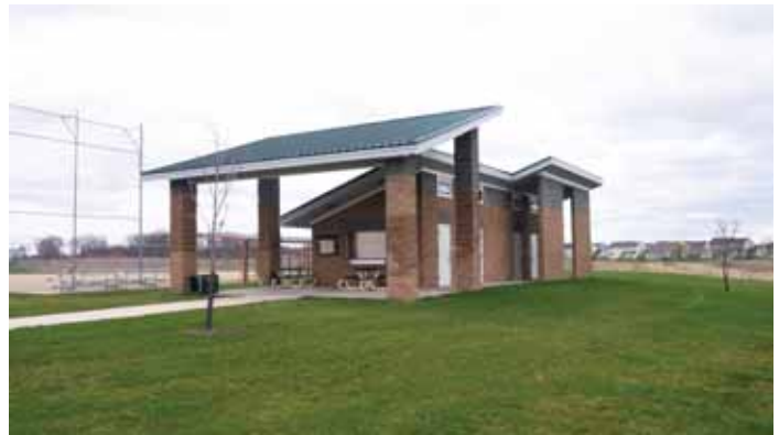
Image 6: Concessions and restroom facilities provide support to the athletics fields on the west site.
