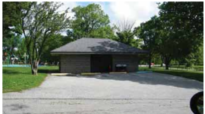
Image 2: The restrooms support extended resident visits to the park facility.
