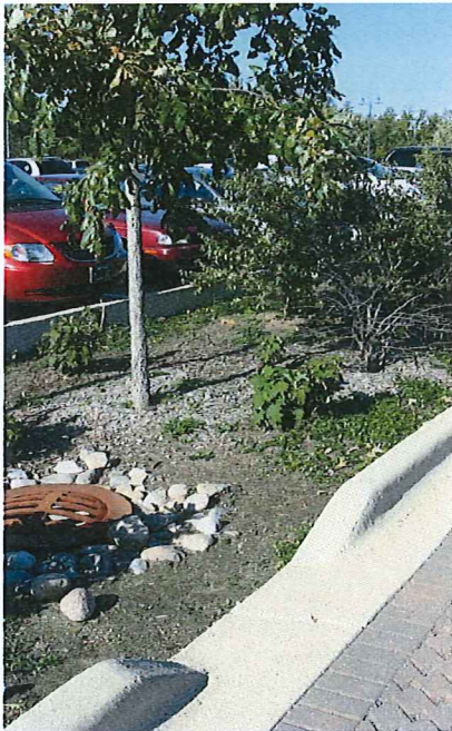
Bioswales are sustainable storm water management systems designed to remove pollutants from surface water runoff. These landscape elements can be used as buffers around parking areas in commercial centers, as well as along streets.
