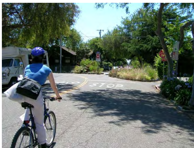
Figures 61 and 62: Traffic diverters allow through bicycle traffic while dispersing motor vehicle traffic onto adjacent roadways.
