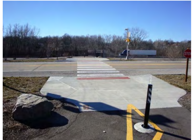
Figure 97: Bollards, ADA compliant curb ramps, high-visibility crosswalk markings, and rectangular rapid flashing beacons help improve user safety at this street crossing.
