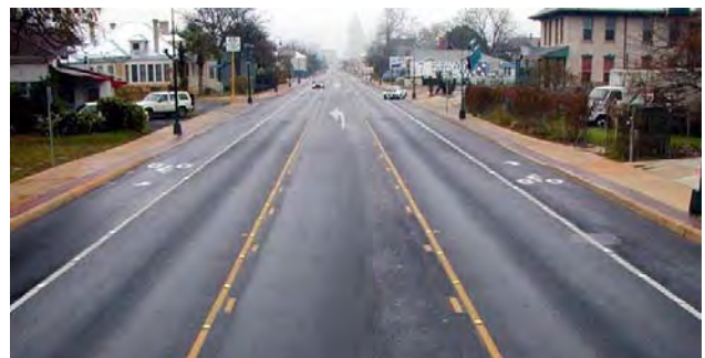
Figures 58 and 59: Before and after images from this road diet show how roadway space can be reallocated to increase space for bicyclists.
