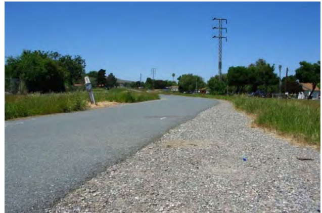
Figure 91: Decomposed granite or crushed limestone can provide an excellent shoulder to meet clearance requirements and provide a desirable surface for walkers and runners.
