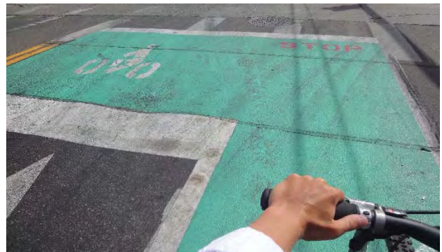
Figure 78: Bike boxes allow bicyclists to proceed through the intersection before motor vehicles.
