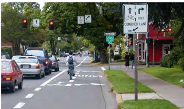
Figure 80: Where width is insufficient to provide a separate bike lane, providing a shared bike and right-turn-only lane can also be acceptable.
