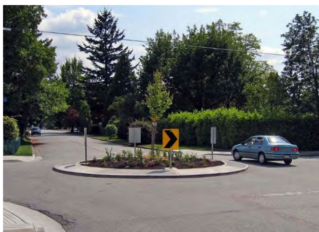
Figure 43: Traffic circles have proven to be effective intersection treatments for bicycle boulevards.
