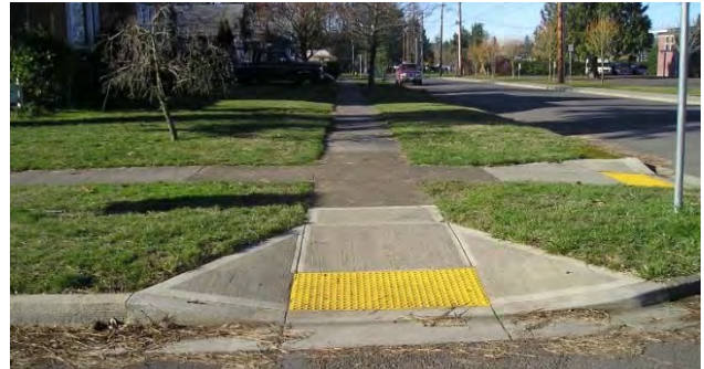
Figure 76: ADA-compliant curb ramps assist persons with physical disabilities in detecting, approaching, and crossing streets.
