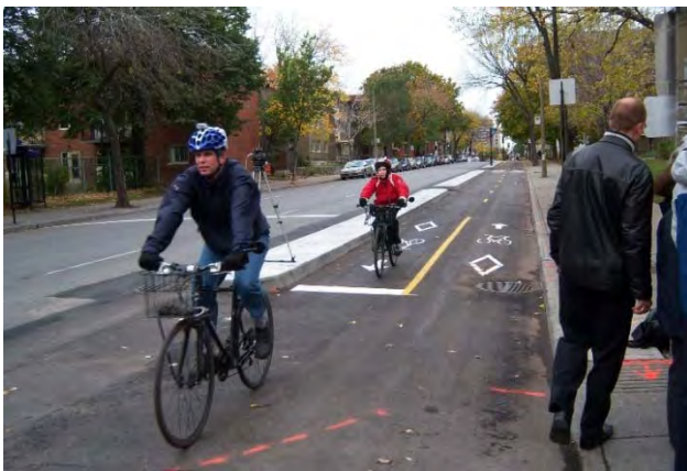
Figure 53: This two-way cycle track is separated from motor vehicle travel lanes by a raised concrete barrier.
