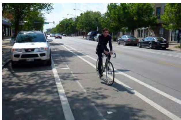
Figure 51: Buffer zones can be provided on both sides of the bike lane, increasing separation from both parked and traveling motor vehicles.
