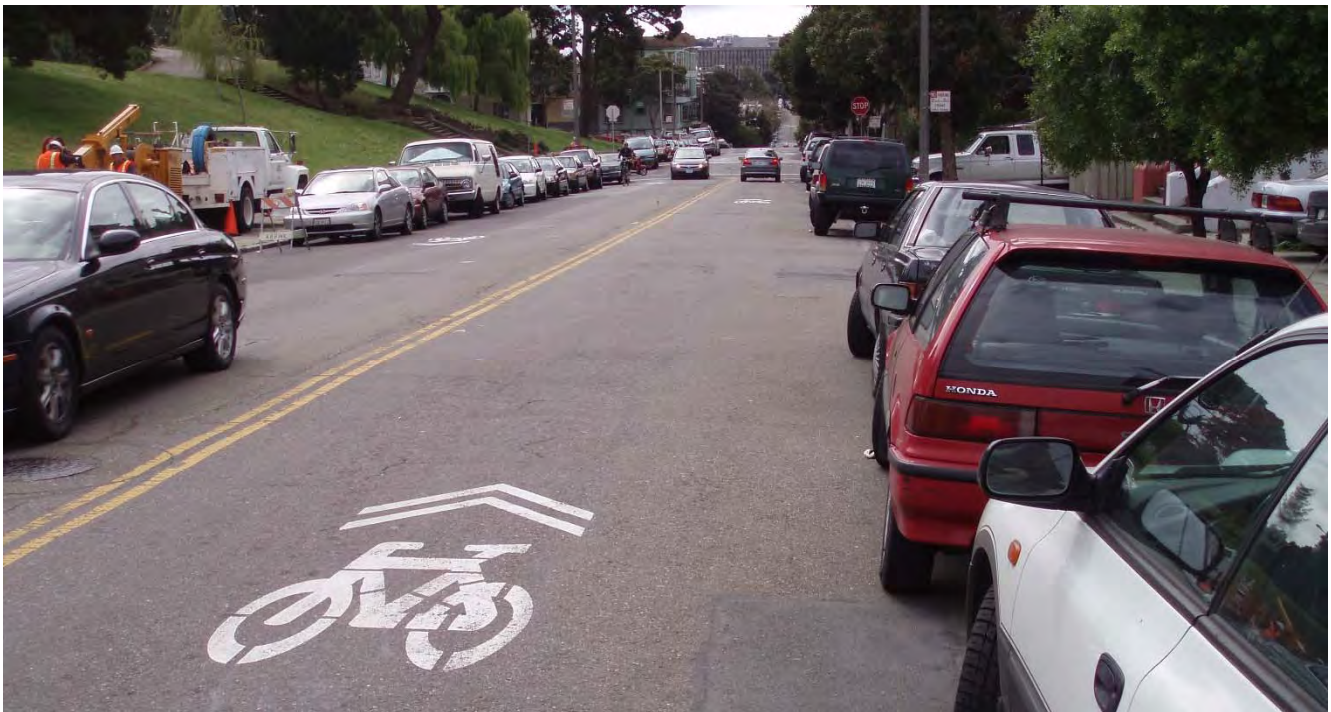
Figure 112: Shared lane markings raise motorists' awareness that the road they are driving on is a preferred corridor for bicycle travel.
