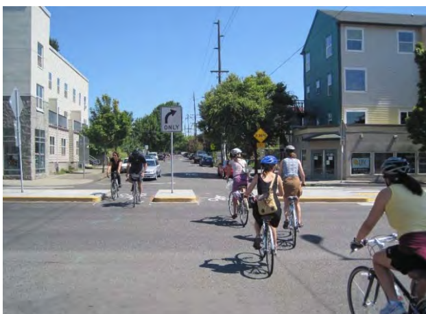
Figure 44: Traffic diverters allow through bicycle movements while restricting motor vehicle traffic.
