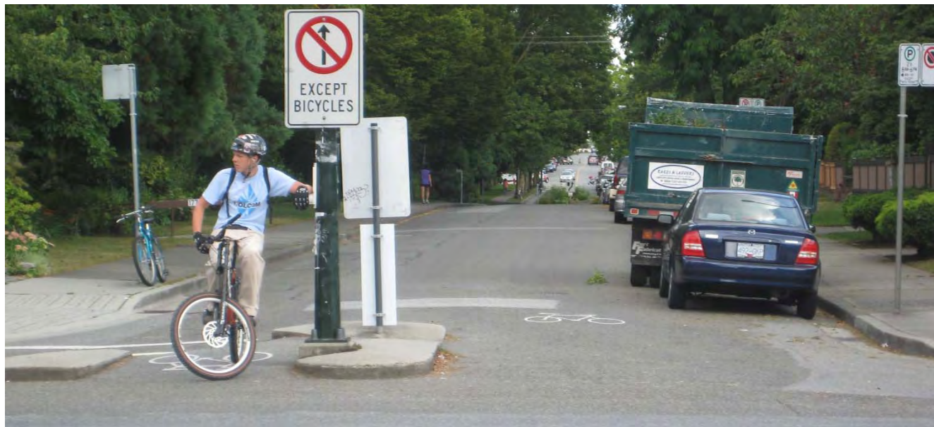
Figure 111: This bicycle boulevard example incorporates traffic diversion elements to reduce through motor vehicle traffic.
