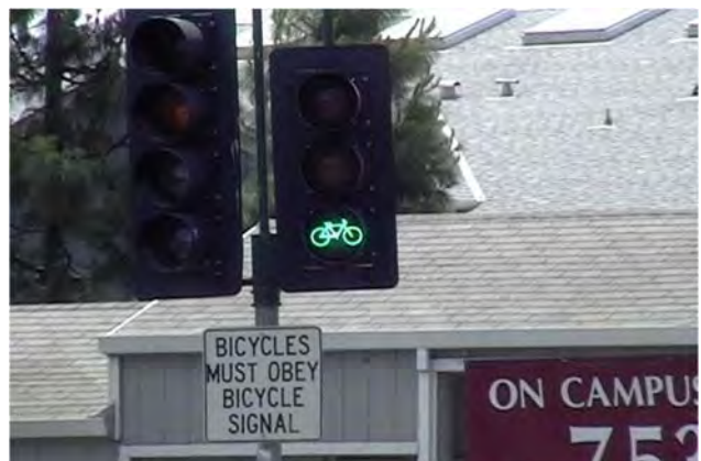
Figure 84: Bicycle signal heads can be used to allow bicyclists to clear the intersection before motor vehicles receive a green light.
