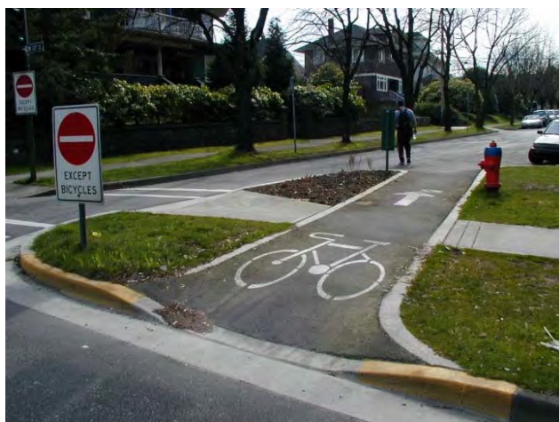
Figures 61 and 62: Traffic diverters allow through bicycle traffic while dispersing motor vehicle traffic onto adjacent roadways.
