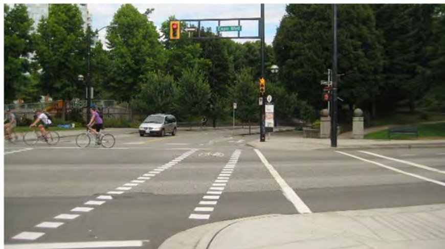
Figure 81: Bike lane markings inside the intersection box increases bicyclist predictability.
