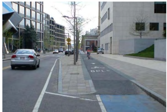
Figure 52: A raised cycle track in Cambridge, Massachusetts.
