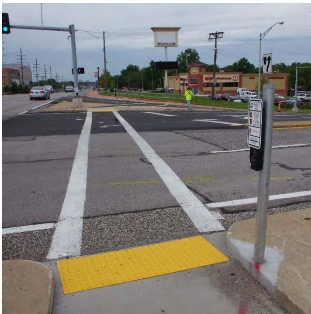
Figure 34: Push button-activated crosswalks and pedestrian signal heads encourage pedestrian compliance at larger intersections.
