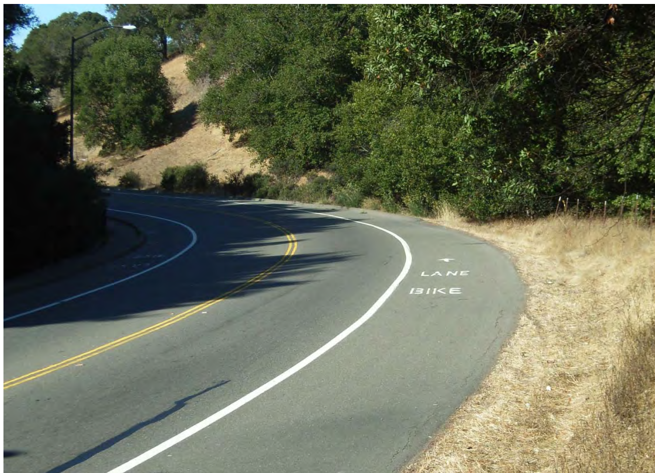
Figure 113: A shoulder bikeway can provide an adequate facility for bicyclists while also serving as a break down lane for motor vehicles.
