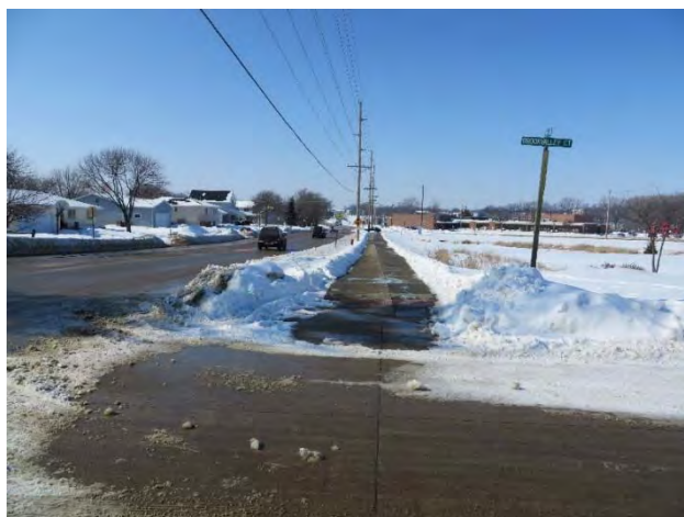
Figure 26: This trail crossing at 29th Avenue and Brookvalley Court lacks any signage, striping, or pavement markings to indicate the presence of the trail.
