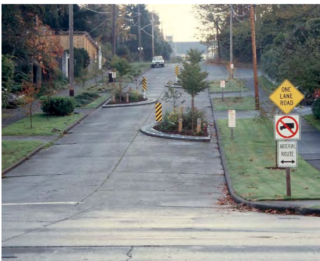
Figures 64 and 65: Chicanes slow motor vehicle traffic, creating a more calm and welcoming environment for both bicyclists and pedestrians.
