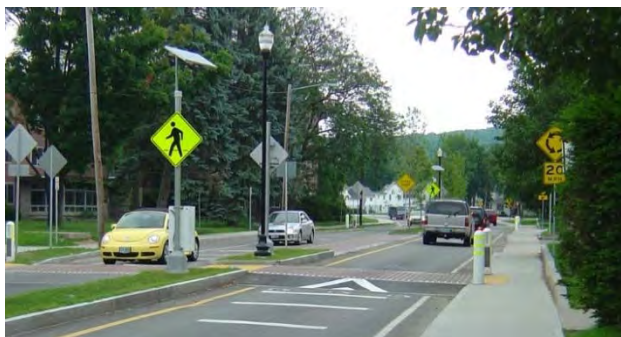
Figure 42: A raised crosswalk doubles as a speed table to reduce motor vehicle speeds.
