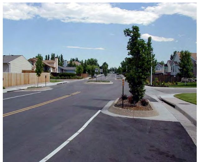
Figures 64 and 65: Chicanes slow motor vehicle traffic, creating a more calm and welcoming environment for both bicyclists and pedestrians.
