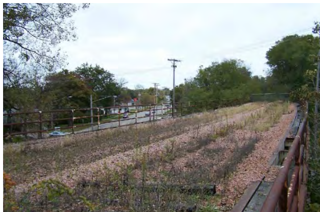
Figure 22: The abandoned rail corridor travels over 7th Street, Marion Boulevard, and Indian Creek via three separate bridge structures (Photo credit: Terri Thayer).
