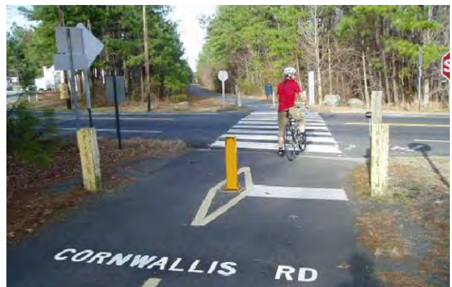
Figure 98: At unsignalized trail crossings, high-visibility crosswalk markings increase motorist awareness of crossing pedestrians.
