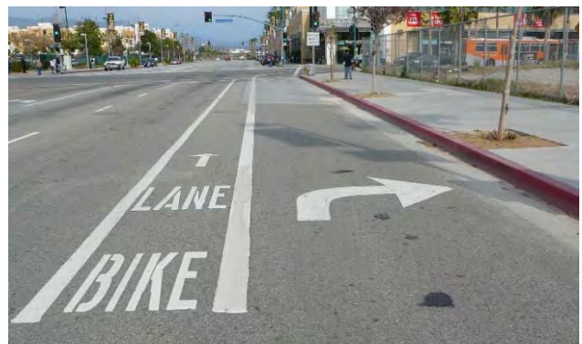
Figure 77: Bike lanes parallel to right-turn-only lanes help to reduce conflict between bicyclists and motorists.
