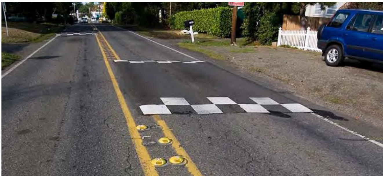
Figure 60: A speed table can effectively reduce motor vehicle speeds, increasing bicycle and pedestrian safety.
