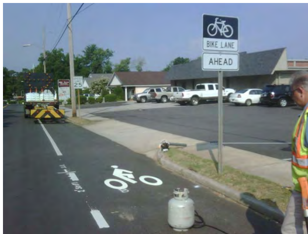
Figure 128: A street crew adds new bike lane markings after a resurfacing project.
