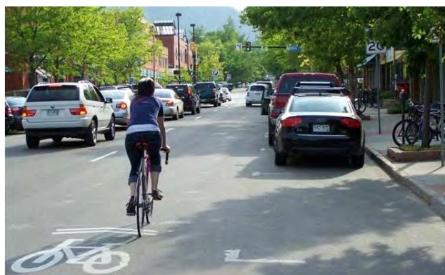
Figure 38: Shared lane markings help cyclists position themselves within the travel lane.
