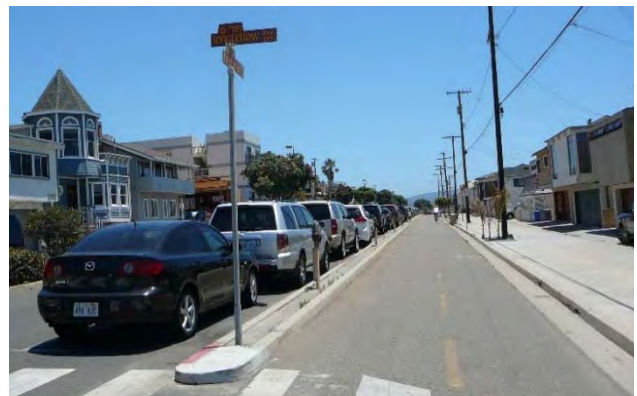
Figure 54: A raised concrete barrier and vehicle parking create adequate separation to provide cyclists with a comfortable facility.
