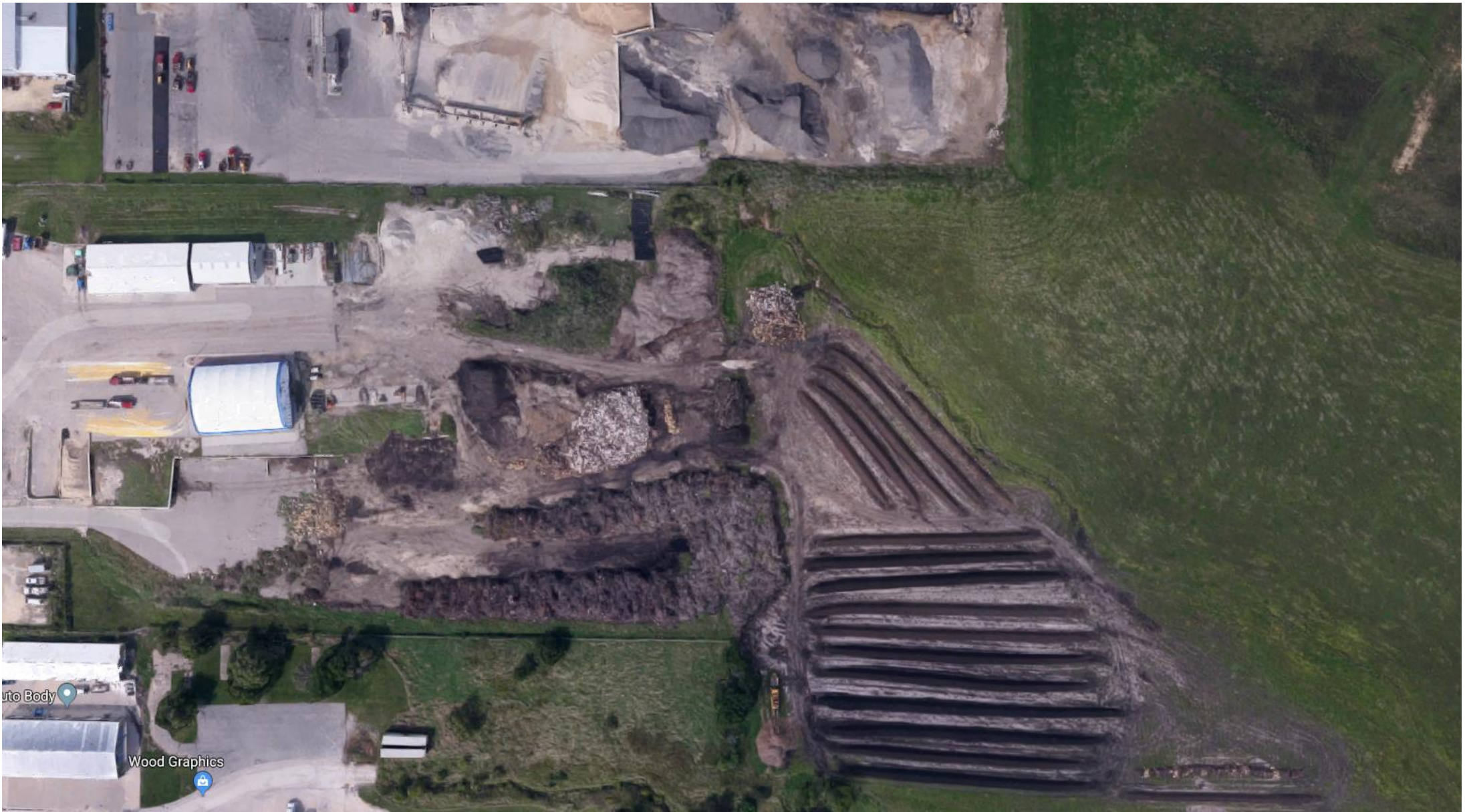
YARD WASTE FACILITIES AT PUBLIC SERVICE 2017
