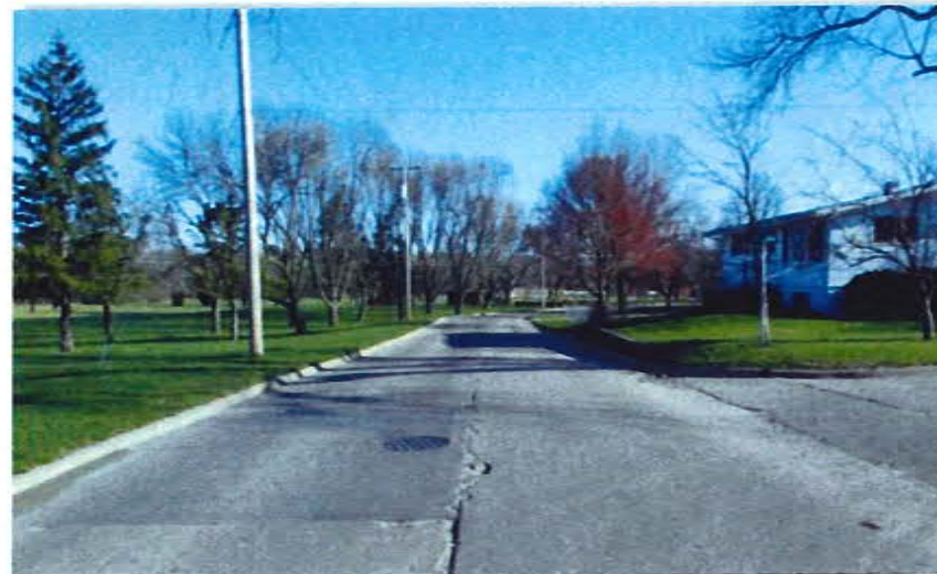
Figure 5: 2nd St at 9th Ave Intersection
