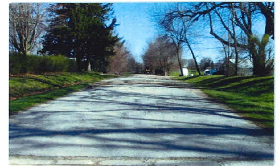
Figure 7: Alburnett Rd north of Boyson Rd
