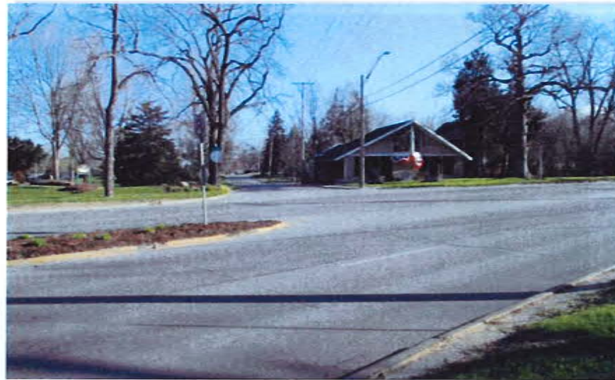
Figure 9: 7th Ave and 2nd St Intersection
