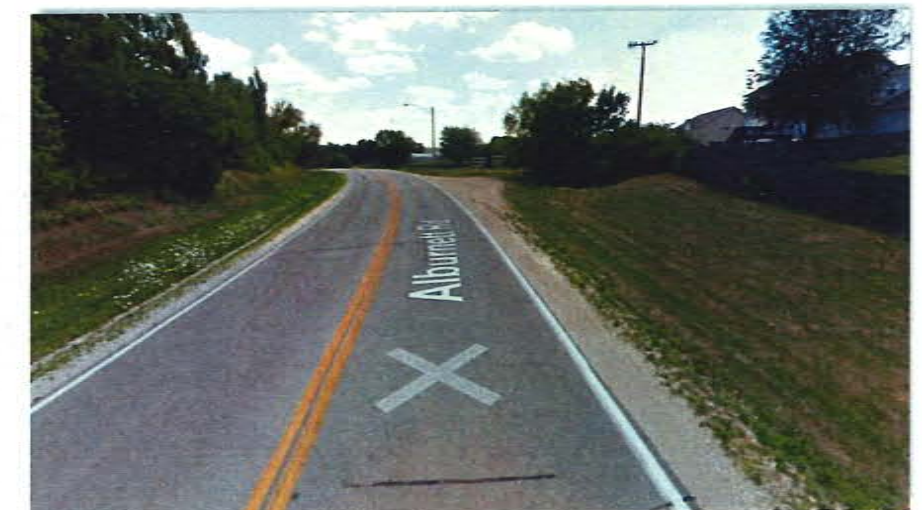
Figure 8: Alburnett Rd at north Project Limits
