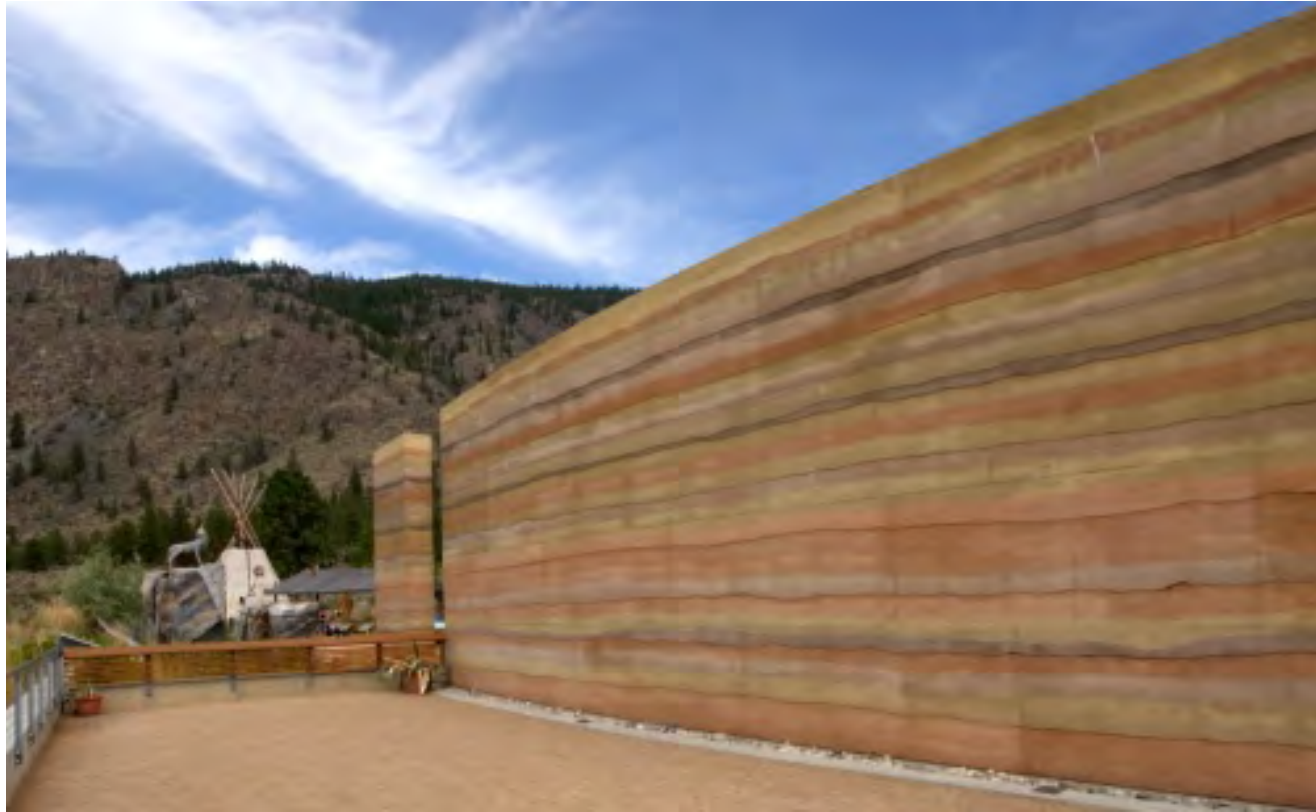
RAMMED EARTH WALL
