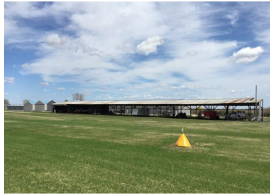
This hangar shed has been removed
