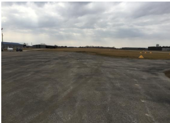
Existing apron looking south
