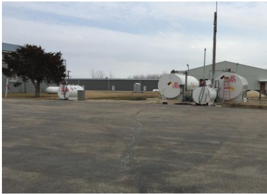
Existing fueling station
