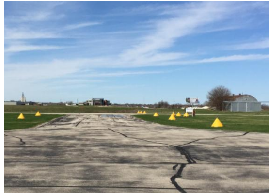
Existing apron looking northwest
