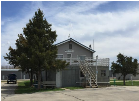
Old FBO Building
