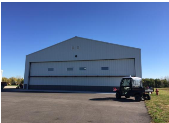
New Maintenance Hangar
