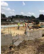
The Marion Water Department has hired WRH, Inc. from Amana to construct a \$2.87 million Iron Removal Treatment Plant at 2351 31st Street. This new facility will be capable of treating 1500 gal/min of water from both the Jordan and Silurian Aquifers to meet the community's future drinking water needs. Construction is underway with work expected to be completed by June 2022.
