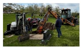
**Cemetery:** Grounds staff assisted in a site opening for a burial after discovering there was a large amount of rock in the location. Staff utilized a backhoe with a hydraulic breaker to break apart the rock so it could be removed. (photo left)
