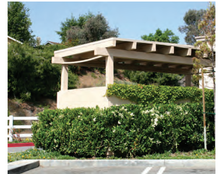
SCREENED TRASH ENCLOSURE
