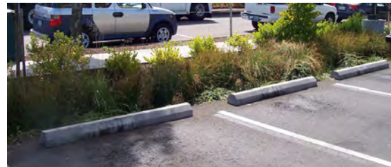
BIOSWALE AT PARKING LOT
