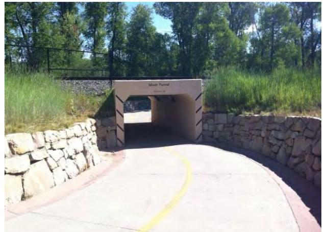
Figure 102: Trail underpasses separate trail users from motor vehicle traffic and/or rail traffic, reducing delays for all users.
