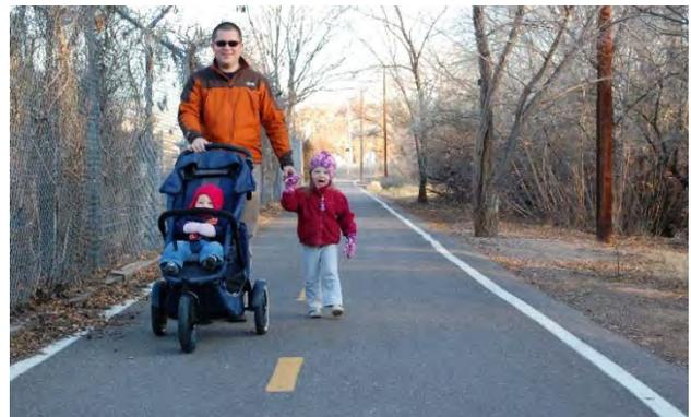
Figure 92: Some shared use paths incorporate both centerline and edge striping.
