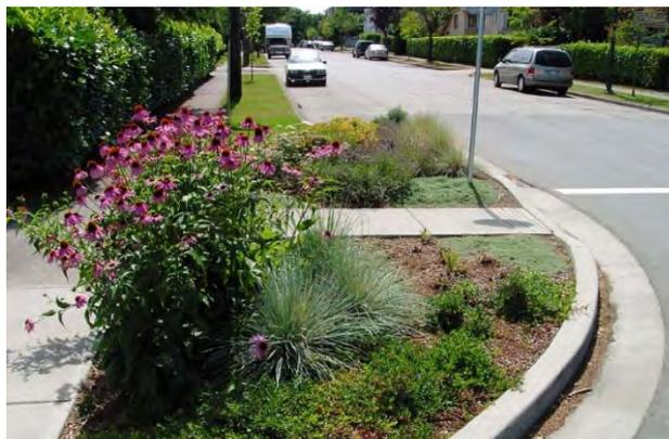
Figure 45: Curb extensions reduce turning radii and shorten pedestrian crossing distances.
